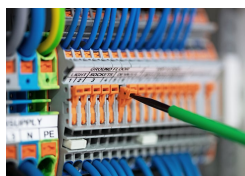
Pivoting a knife disconnect.
