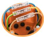
Wiring conductors in a flush-mounted junction box.
